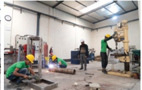
Supervision on panel fabrication
